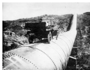
This is the original Los Angeles aqueduct, bringing water from the Owens Valley all the way to LA. This one was built of iron. In the 1970's, another smaller aqueduct was built of steel.
